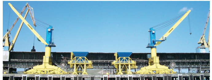
BulkLogisticLandmark was involved in the upgrade of the Toros Ceyhan terminal
